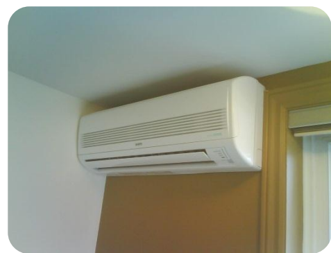
Indoor unit of a split air-conditioner
