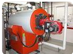
Condensing boiler
